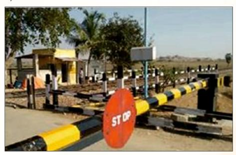
RITES always checks & compares the extent of lifting of an electrical lifting barrier through electric excitation vis-à-vis the lifting when done through hand-cranks.
