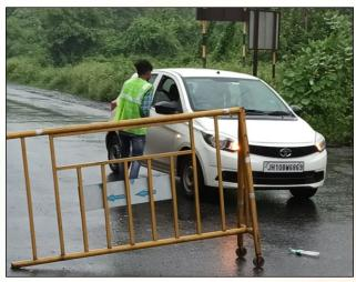
Survey team wears retroreflective gears and ensures traffic control devices like barricades and speed barriers are installed at survey locations.
